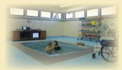
The Solo-Step Track System consists of a high-performance, overhead aluminum track and trolley mounted to the ceiling. An attached harness protects patients from falling, which helps instill confidence.
